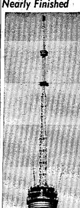
Work on the 220-foot television tower atop the Empire State building in New York is nearly completed as work-men stud weld the conduit strips for the transmission lines that will carry radio and TV programs to the tip to be
